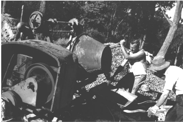
Mixing the Concrete
